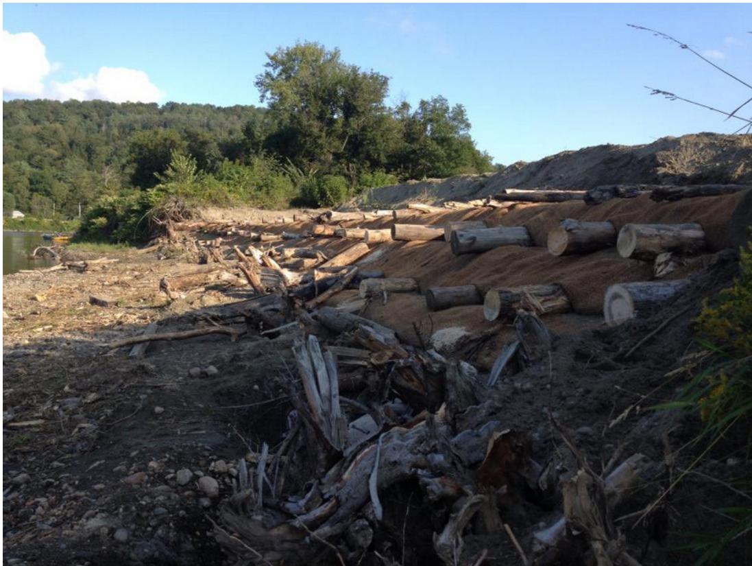
Stage 2 project site in August 2013.
