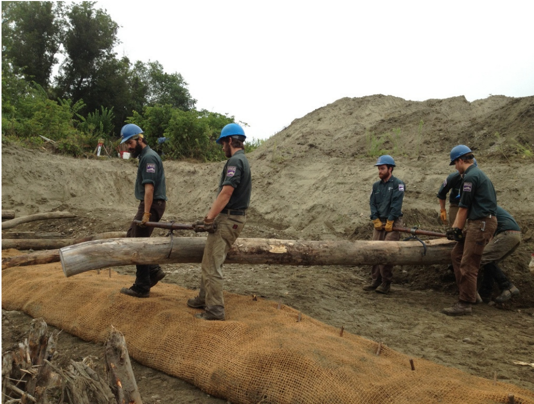
Placing an ice fender on top of a completed soil lift.
