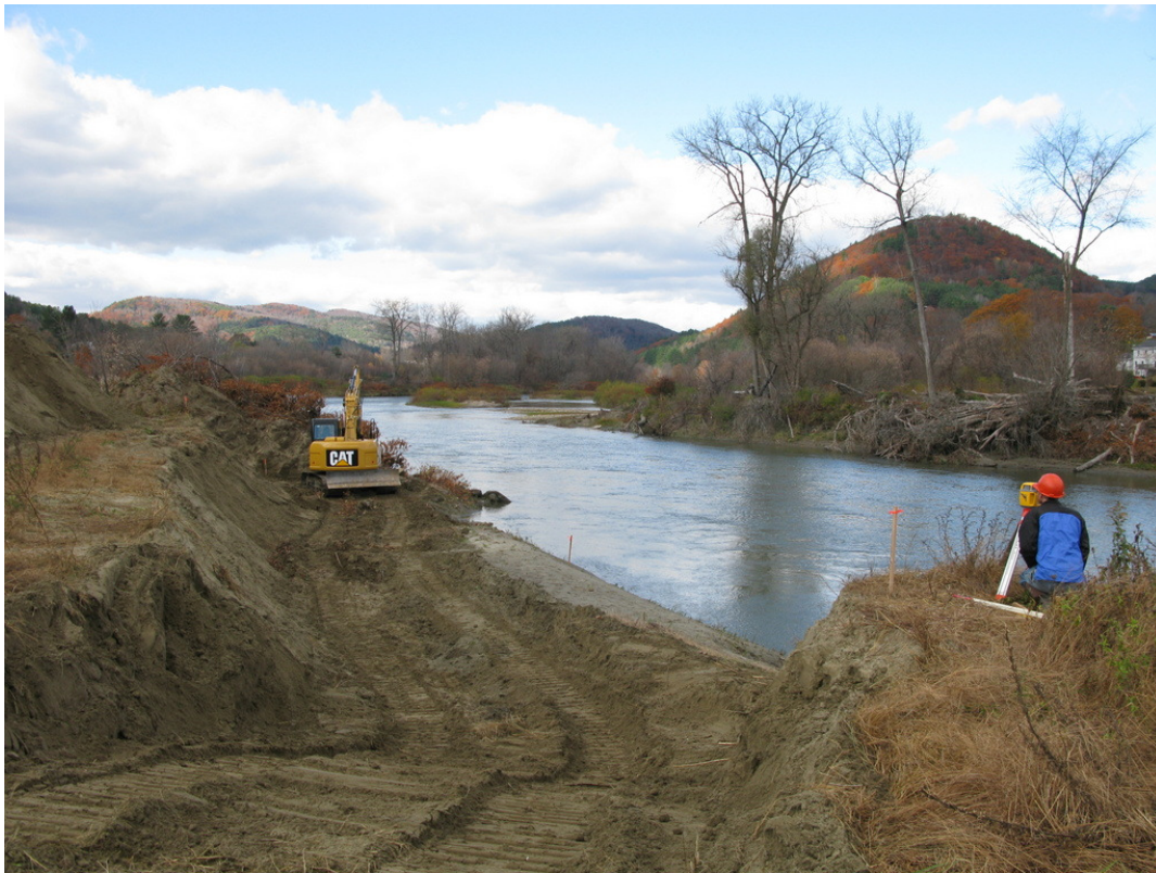
Excavating the upstream project site to the low-water elevation.
