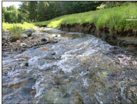
Figure 5.18. Riparian buffers are lacking in T3.2-S3.01-A and bank erosion is abundant.
