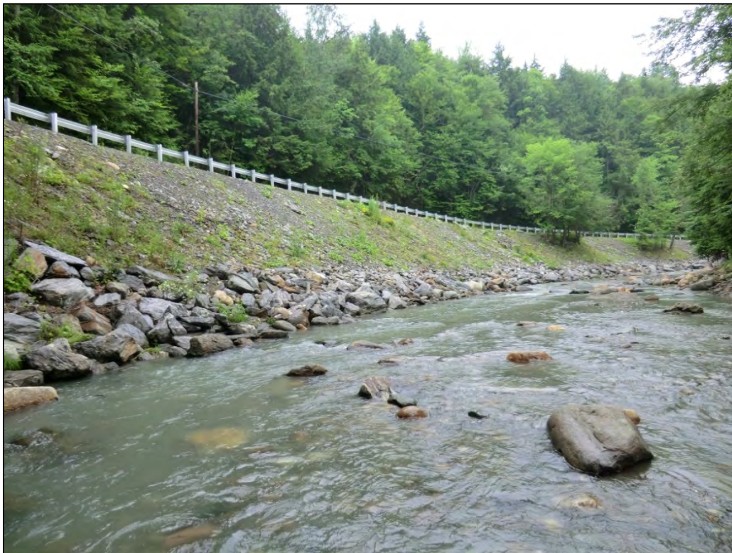
Figure 5.30. Much of T5.01-B was historically straightened along Stony Brook Road and is extremely incised.
