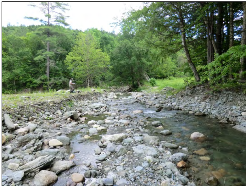
Figure 5.43. Fletcher Brook was extensively dredged and windrowed at the alluvial fan in T5.3-S1.01-A after Irene.
