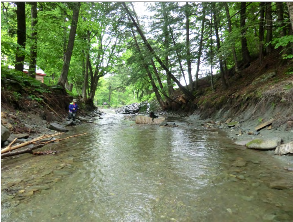
Figure 5.12. Extreme channel incision has occurred and continues to occur in T3.04-C.
