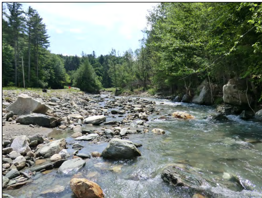
Figure 5.35. Stony Brook avulsed and destroyed a camp and Stony Brook Road in T5.04-B (left side of photo).
