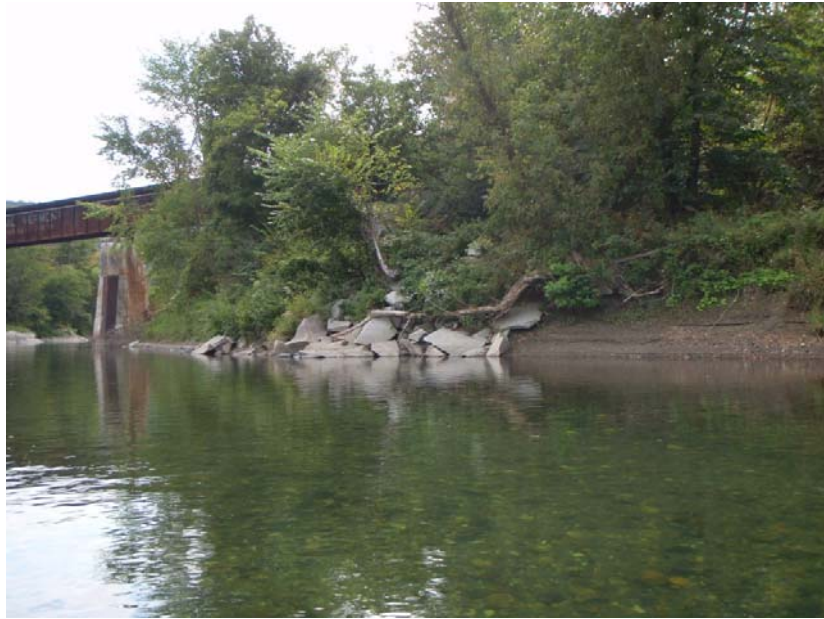
Figure 4.8 Bank erosion and failing rip-rap upstream of the railroad trestle
