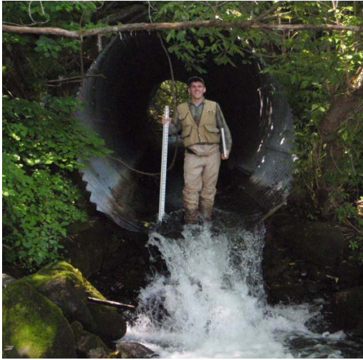
Figure 4.53 A perched culvert at the Route 14 crossing
