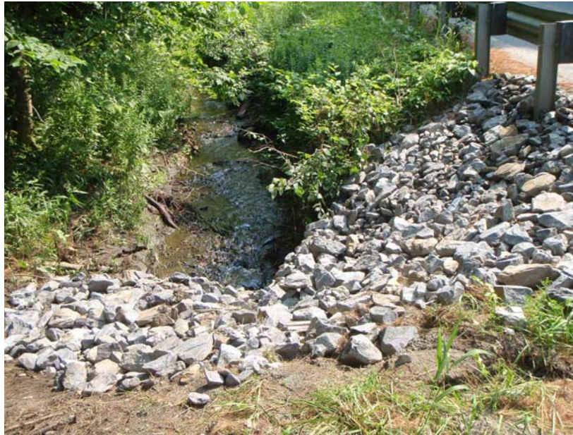
Figure 4.24 Armoring upstream of an undersized culvert (Rt. 132)
