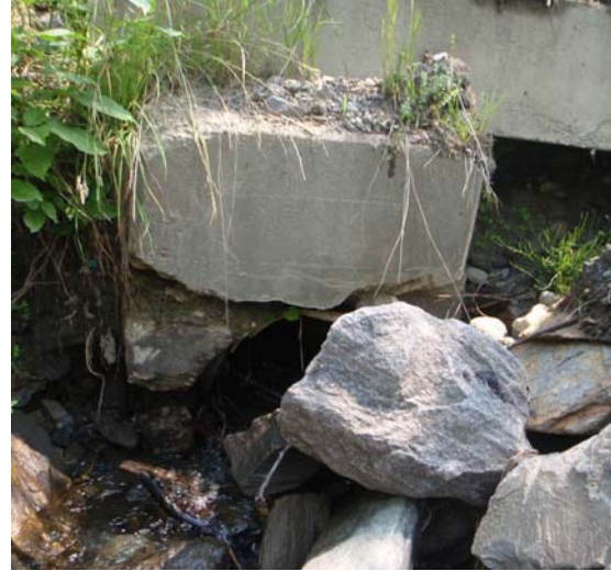
Figure 4.26 Deteriorated outlet of the Cross Road culvert
