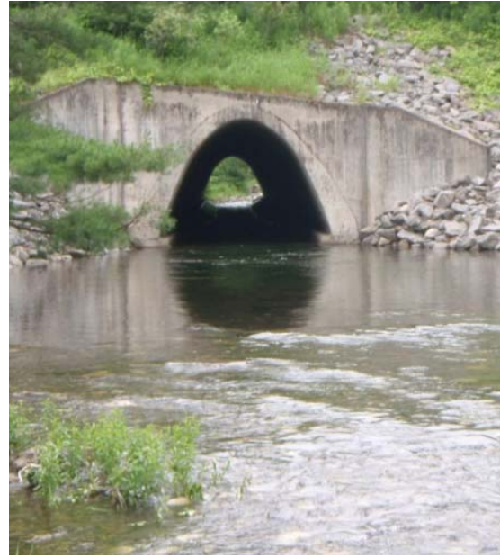
Figure 4.61 Misaligned I-89 culvert with large plunge pool
