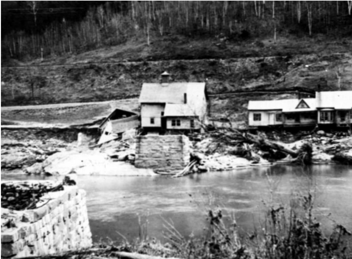
Figure 2.10 The abutments of the washed-out bridge in Sharon; the house was moved downstream (UVM Landscape, 2010)
