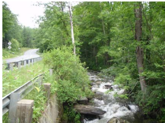
Figure 4.13 Channel encroachment by Rt. 132 and armoring
