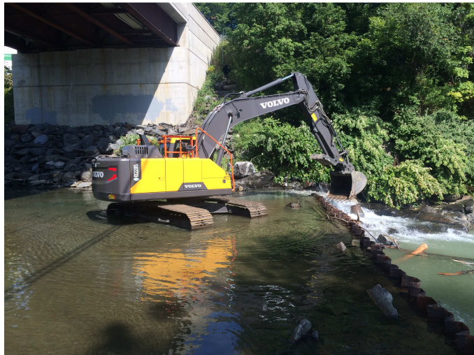
Photo 3: Contractor Ben Canonica removed the sheet pile dam with an excavator
