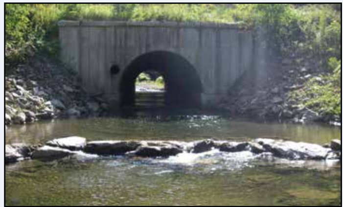
Constructed rock weir eliminates outlet perch.
