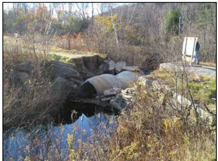
Roadway failure.
