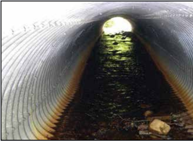
Original corrugated metal culvert.
